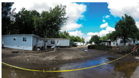
A trailer park in Longmont, Colorado damaged by the September floods.
